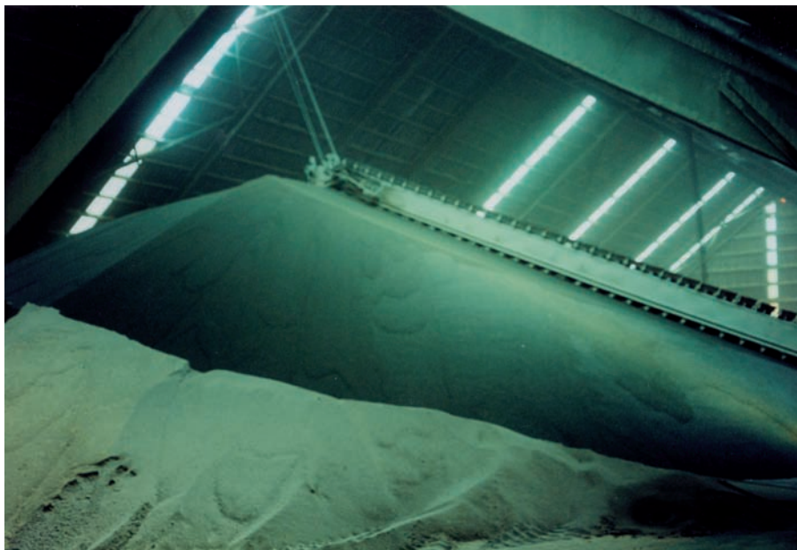
FIG. 1. Dry products storage area.
